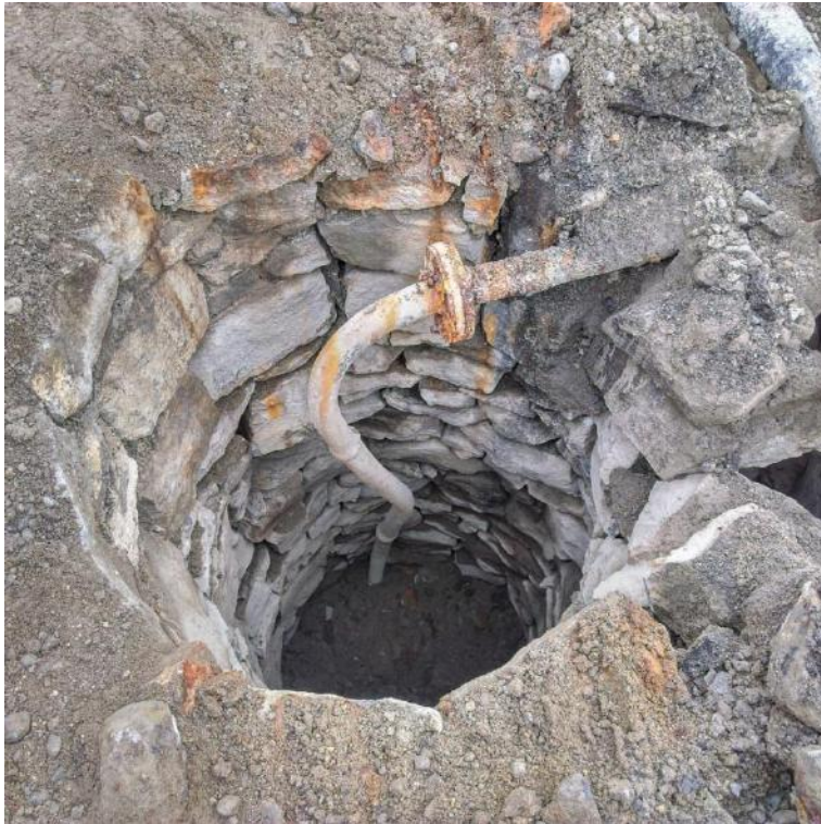
Pl. 9 Well and pump mechanism exposed.
