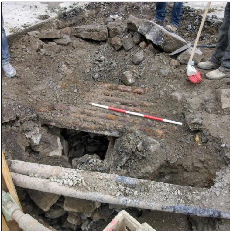
Pl. 8 Cast iron grate across the top of the well opening.
